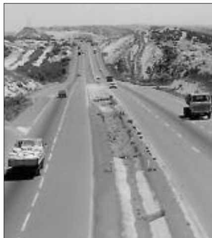
• Five-year plan... New road development is part of the Government's PPP strategy
