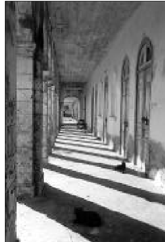
• Cloistered shade at Apostolos Andreas... Soon to be restored to its original condition.
